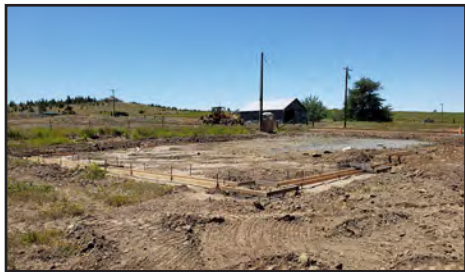
Looking across concrete forms to new power pole
