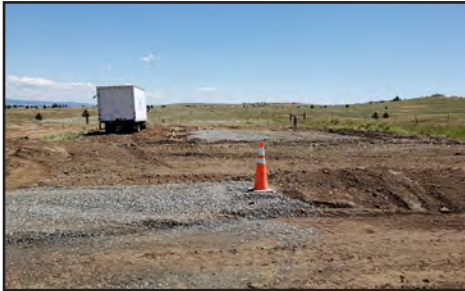
Gravel over new culvert at driveway
